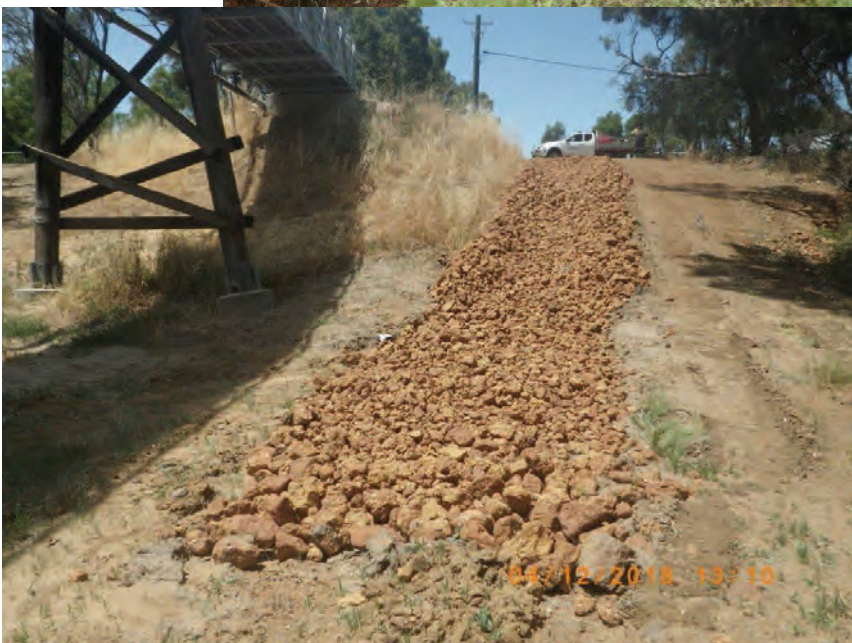
Rockwork to manage erosion. Photo: Greg Warburton, December 2018
